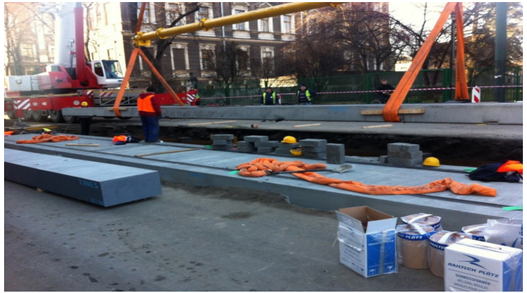
Pic. 7. Laying of the slab TINES LC-L XL.
