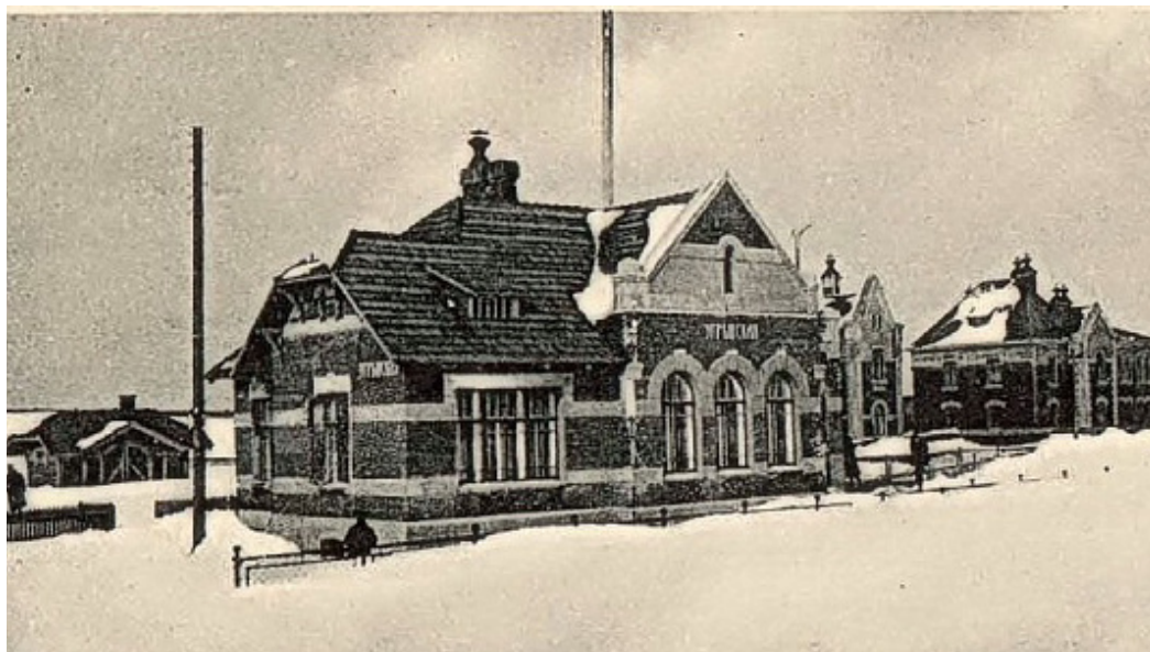
Passenger building at the station Ugreshskaya, 1907.
