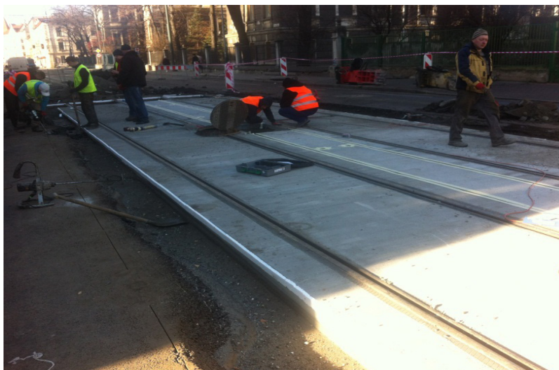
Pic. 10. Installation of polystyrene foam formwork before pouring out the concrete mix.
