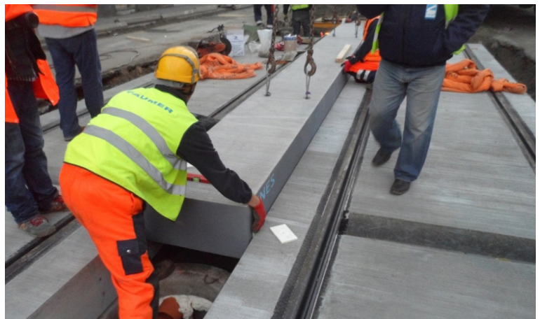
Pic. 9. Laying the plate of the intertrack space in the sewerage area.
