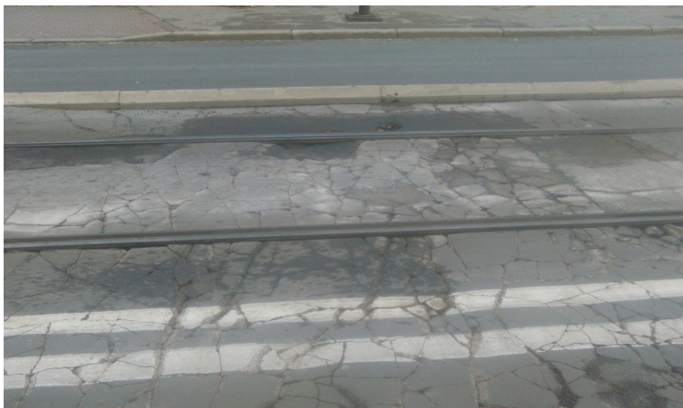
Pic. 1. Significant cracks and chips in the covering.
