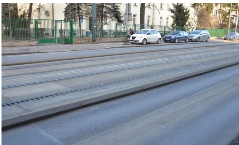
Pic. 11. Rail coating after repair with the system of plates manufactured by the manufacturer TINES LC-L XL.
